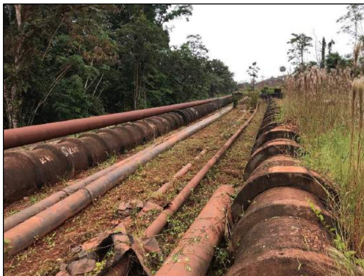
Figure 4.13 Effluent pipes from DRS1, picture facing towards DRS1
