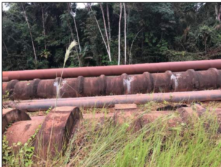
Figure 4.15 Example of small repairs of concrete pipes
