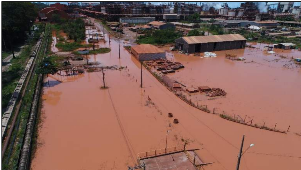
Figure 4.20 Area 45 during the flooding
