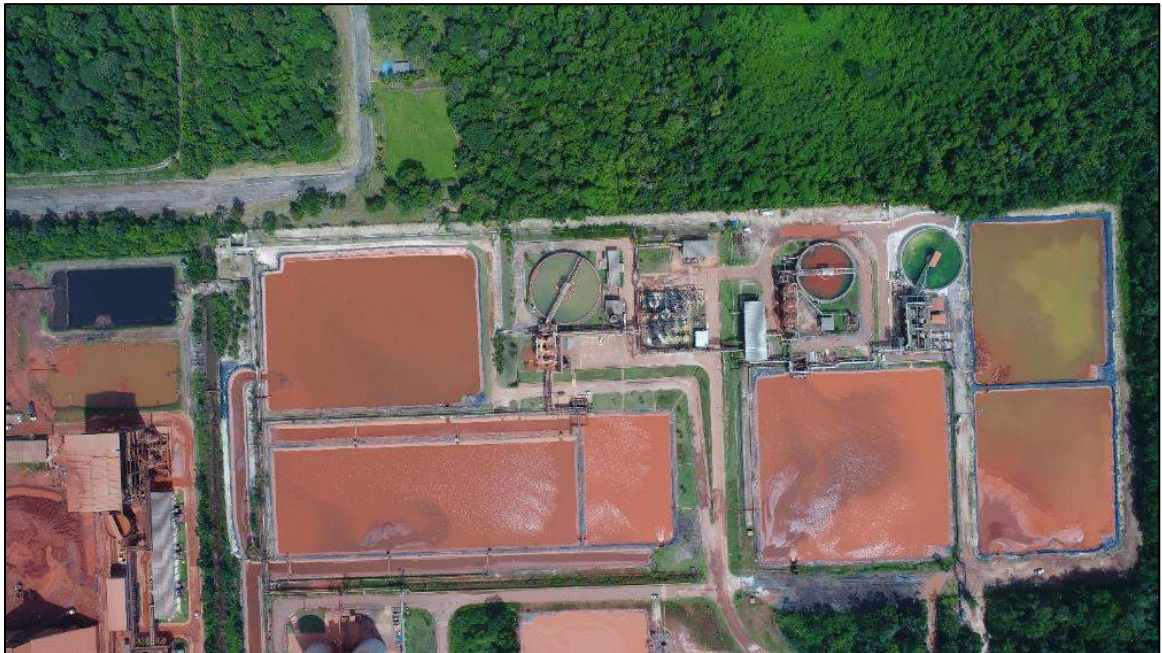
Figure 4.17 Drone photo of Area 82 March 6 th , 2018
